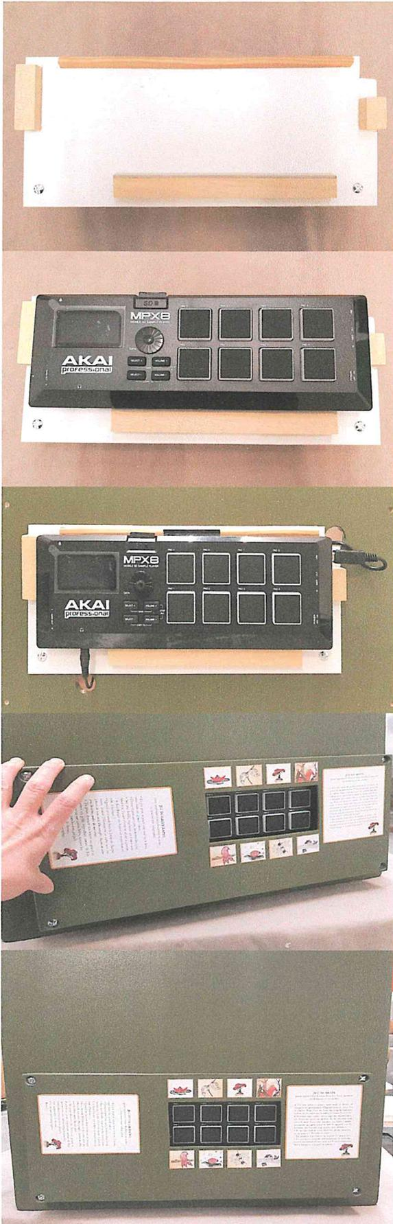
Installer et boulonner le support du sample player MPX8.
